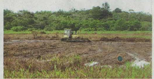
LEVELLING the land for the padi trial planting in Sekuduk-Chupak.
